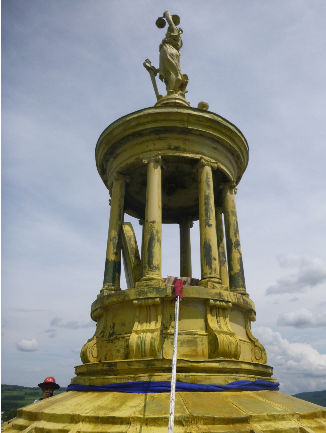
Figure 1: Cortland County Courthouse lantern and top of dome.
