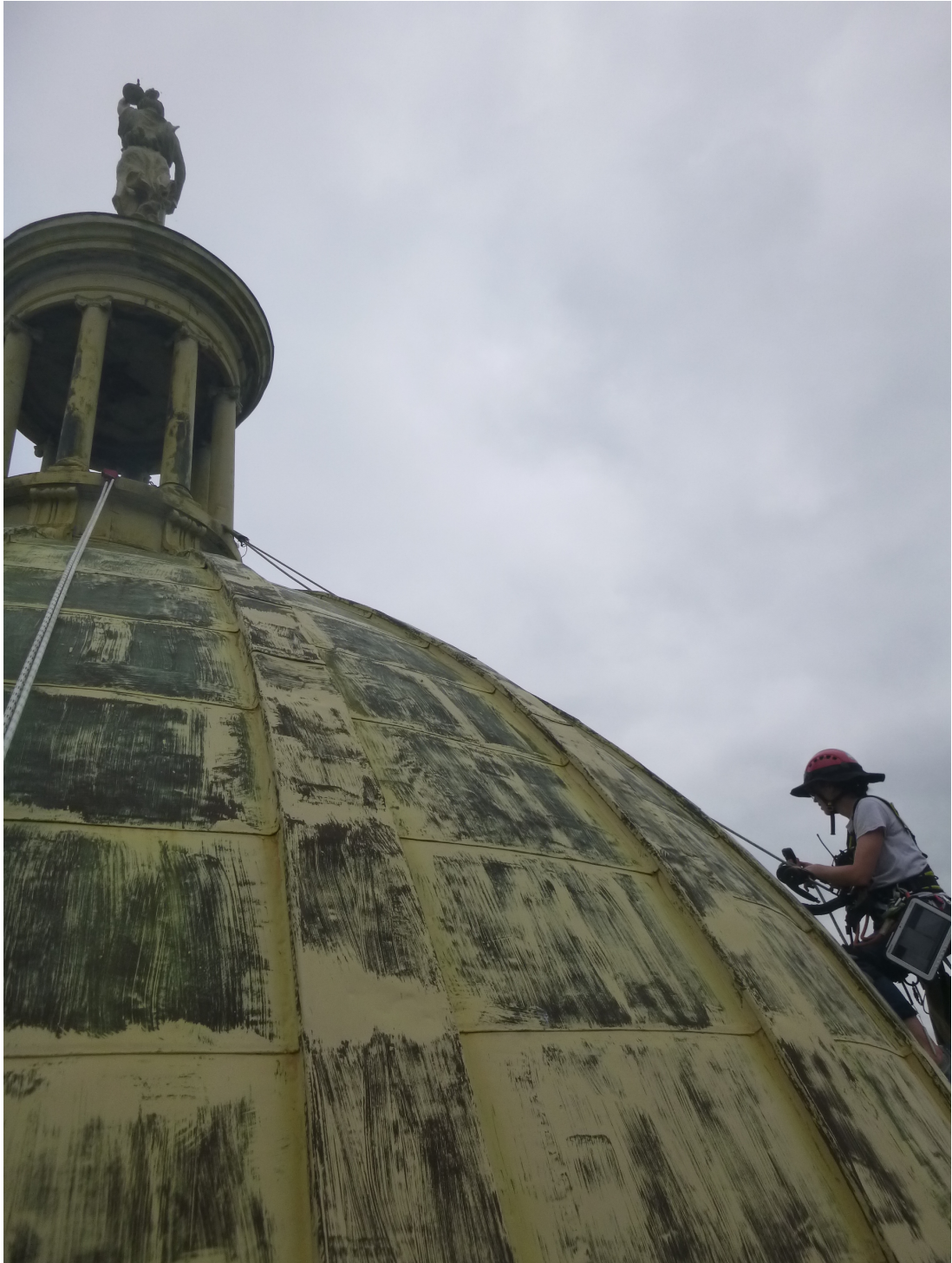
Figure 2: Dome photograph showing pans and rib covers.
