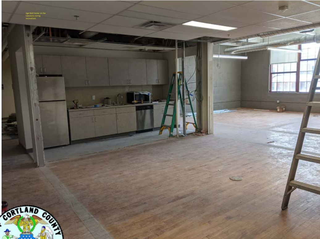
CORTLAND COUNTY AGE-WELL CENTER BEFORE
