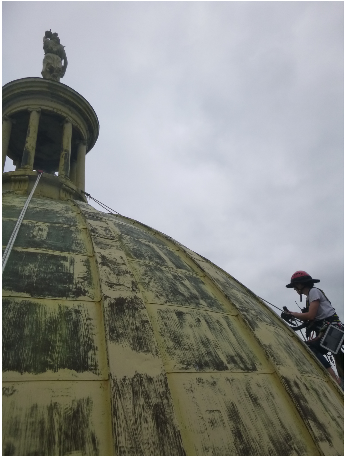
Figure 2: Dome photograph showing pans and rib covers.
