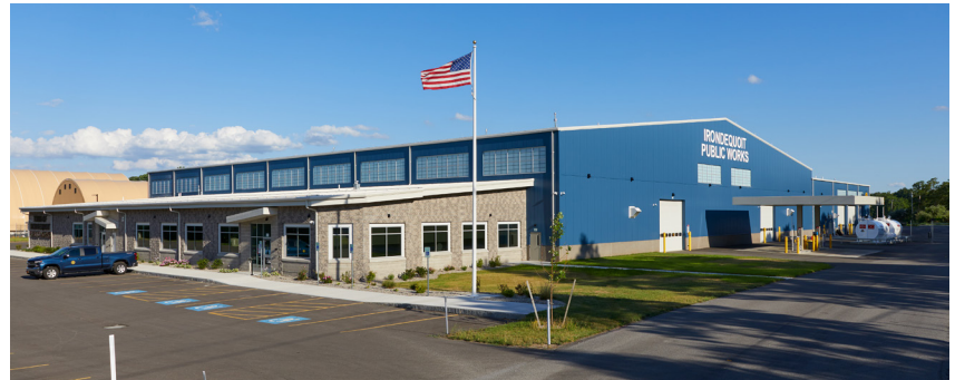
Irondequoit Department of Public Works | Irondequoit, NY
