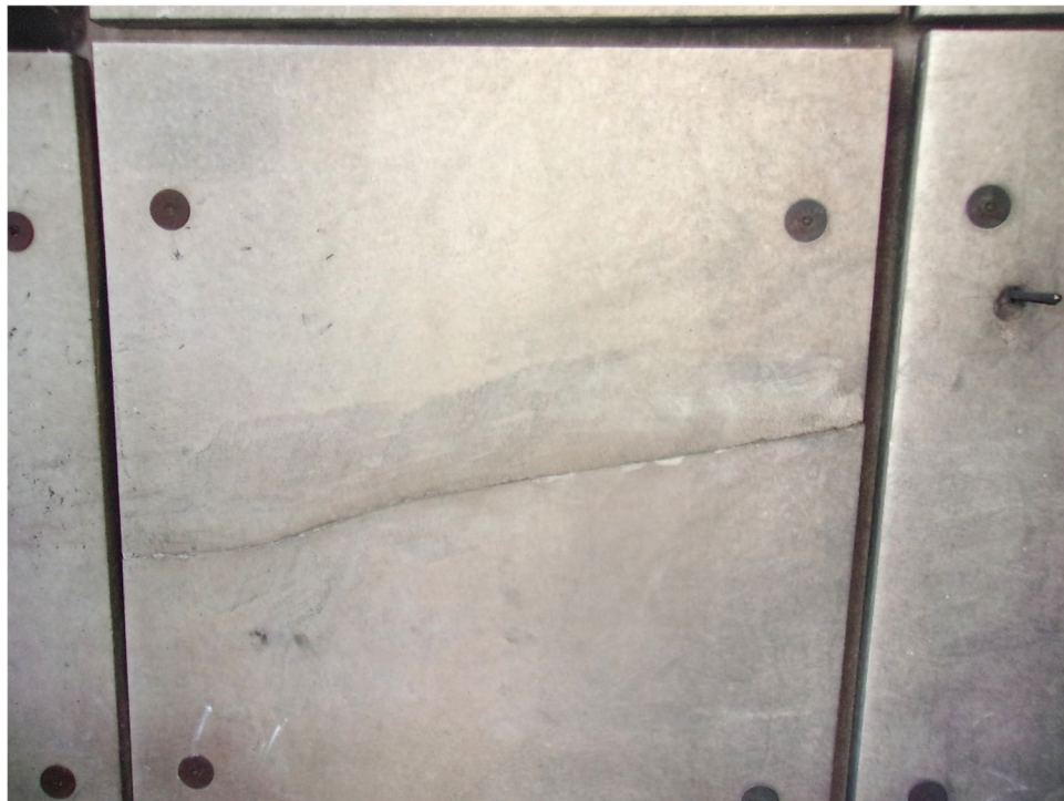
Typical cracked Padgenite panels at burn room ceilings (above) and walls (below)
