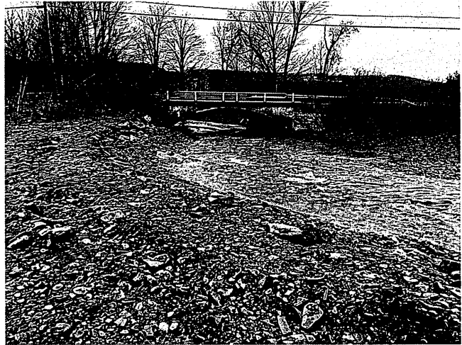
After—Rock riprap installed to stabilize streambanks and minimize erosion. Rock barbs in the stream channel deflect flow and help control gravel.
