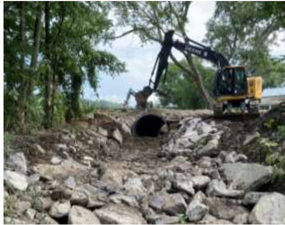
After—Pipe size was increased to improve storm passage. Pipe elevation was lowered to minimize plunge pool at outlet and rock riprap installed to stabilize streambanks and minimize erosion.
