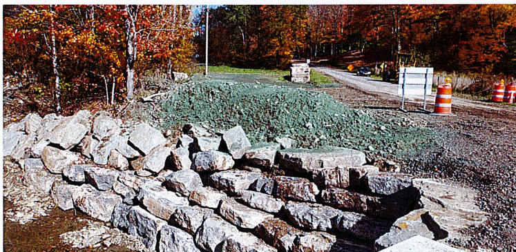
After 2 Bank protection and hydroseeding to prevent erosion.
