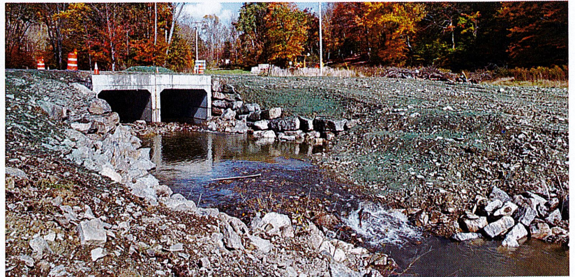
After 1 SWCD negotiated permit conditions and assisted Town with installation of required structures.
