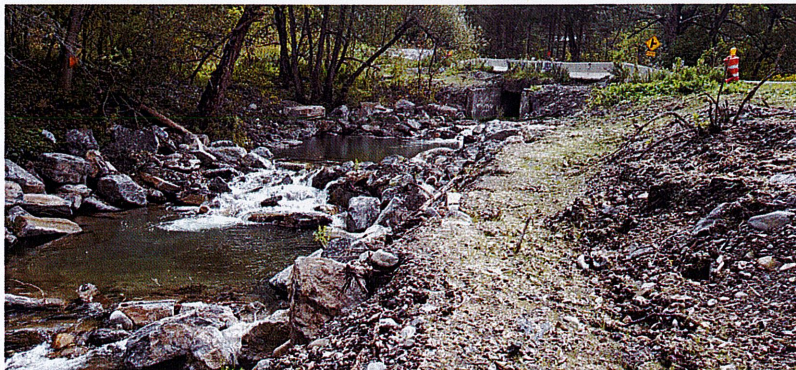
After 1 Bank stabilization, culvert outlet repair for fish passage, corridor stabilization and grade control including low flow channel and flood bench.
